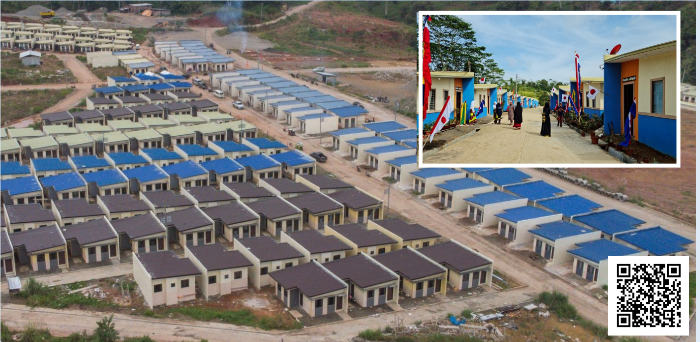
Rehabilitation of Houses in Marawi (Photo: UN-Habitat)
