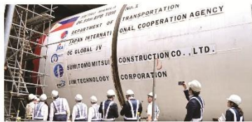
Inspection of the ongoing developments in the Metro Manila Subway Project (MNSP)
