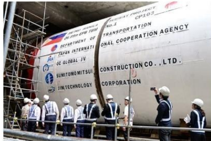
INSPECTION of the ongoing developments in the Metro Manila Subway Project (MMSF).
